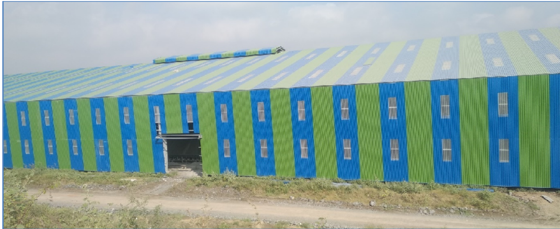
Closed Limestone Storage Shed
