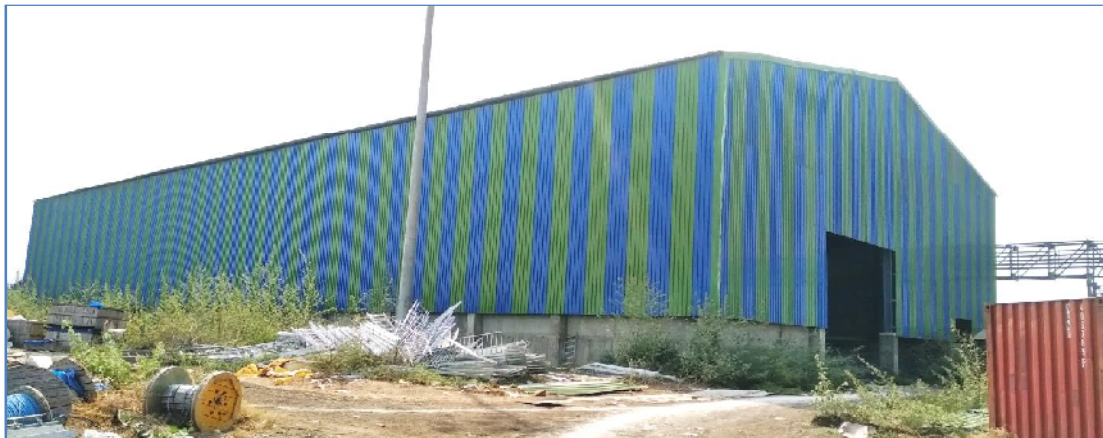
Closed Gypsum Storage Shed
