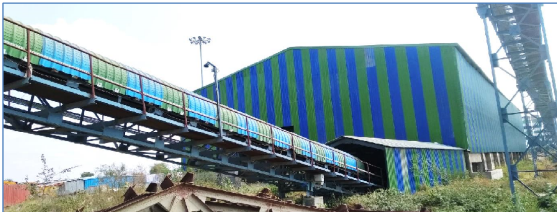
Gypsum storage shed & Closed conveying system
