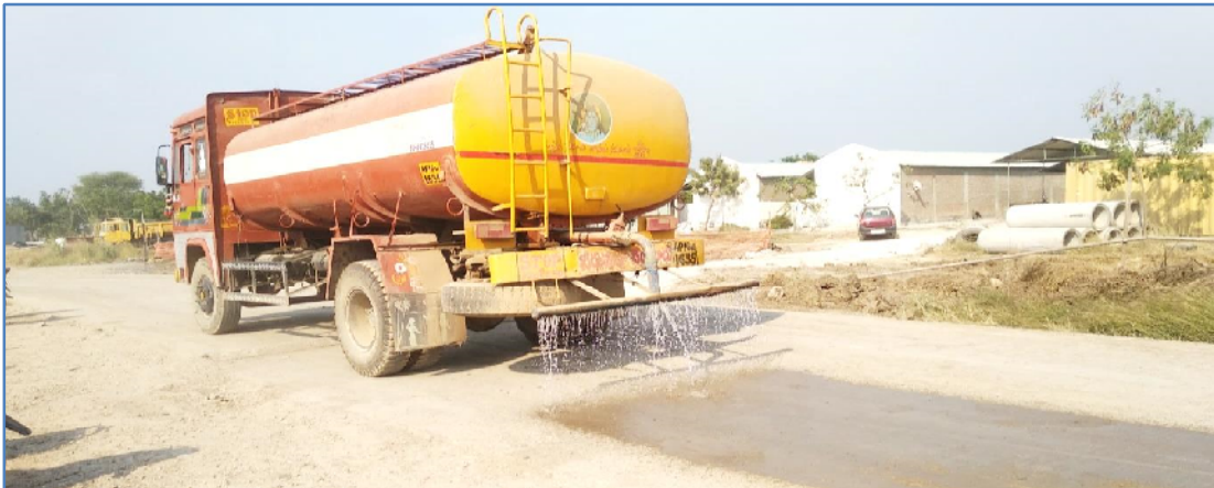
Water spraying on internal roads
